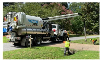
For residents who have had a visit from the VDOT vacuum truck, the next step is to make sure there is a clear and level path from the bottom of your culvert pipe to the next culvert pipe on either side. If the ditch is higher than your cleared pipe, then the water will not flow... clear a narrow path for the water and let nature follow its course. Also, be sure to rake leaves out of the ditches regularly and keep the vegetation in the ditch cut low.
