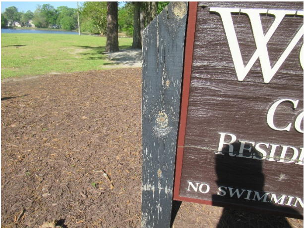
Wood post deterioration
