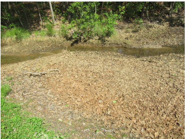
Buildup of sediment and leaves at northeast corner of the pond
