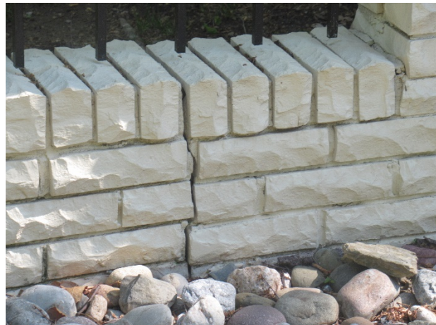
Masonry crack
